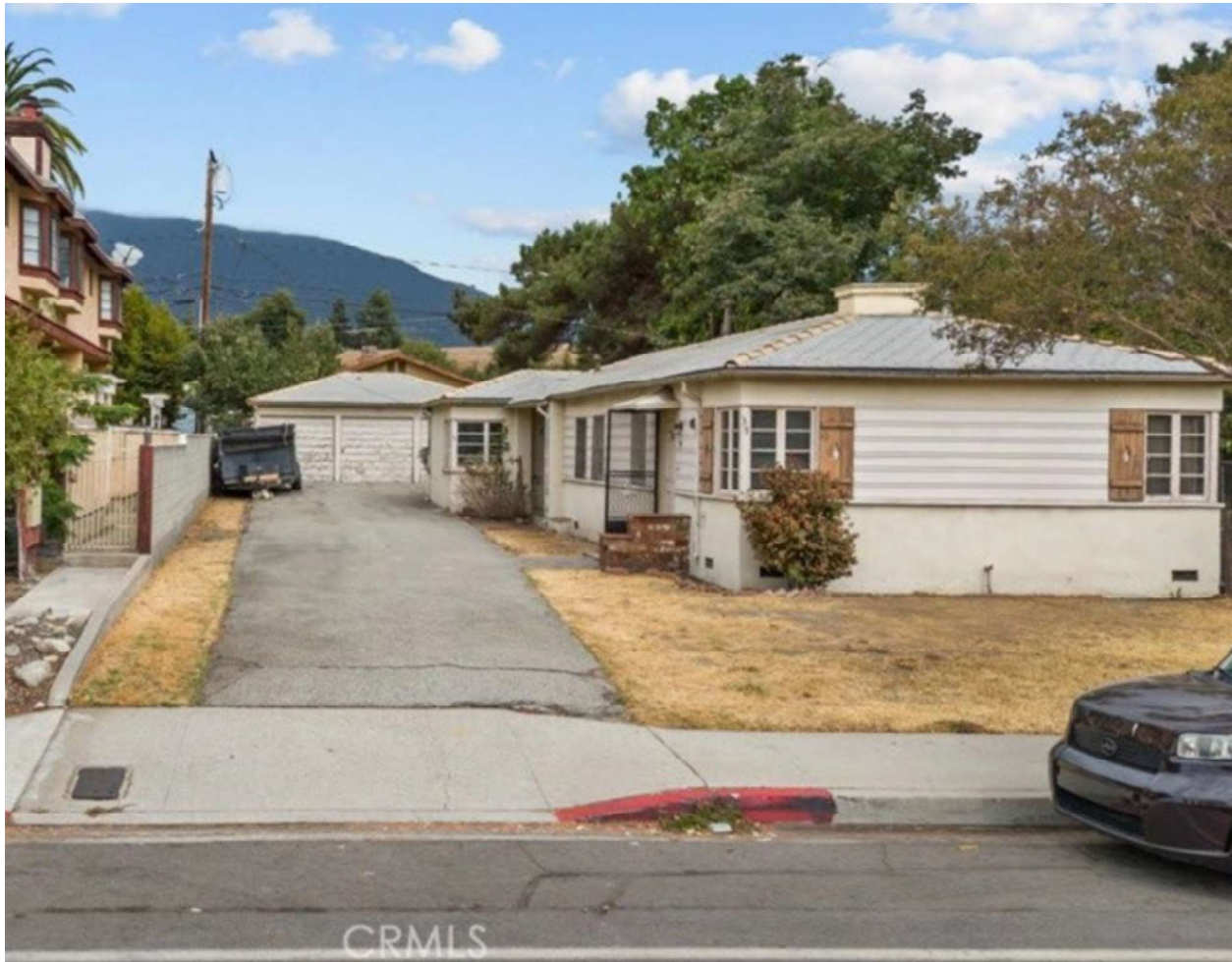
Figure 1 – Subject Site at 33 E. Colorado Blvd.
